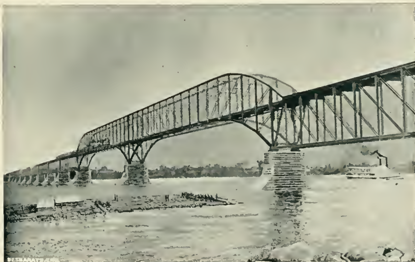
ST. LAWRENCE BRIDGE, C. P. R., LACHINE.
